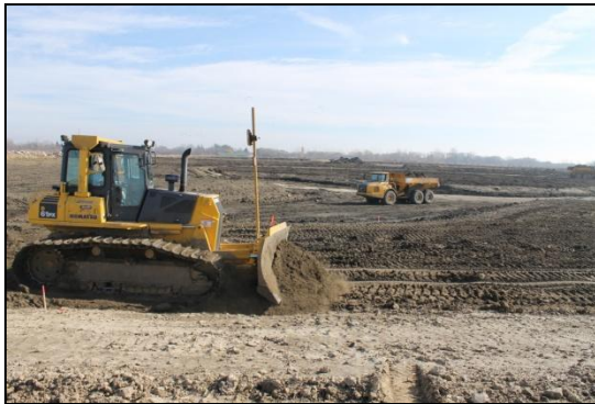
Recontouring of lagoon sludge in Cell 1, October 2012.
